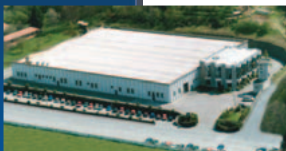
VIR Spa - Valduggia Headquarter
